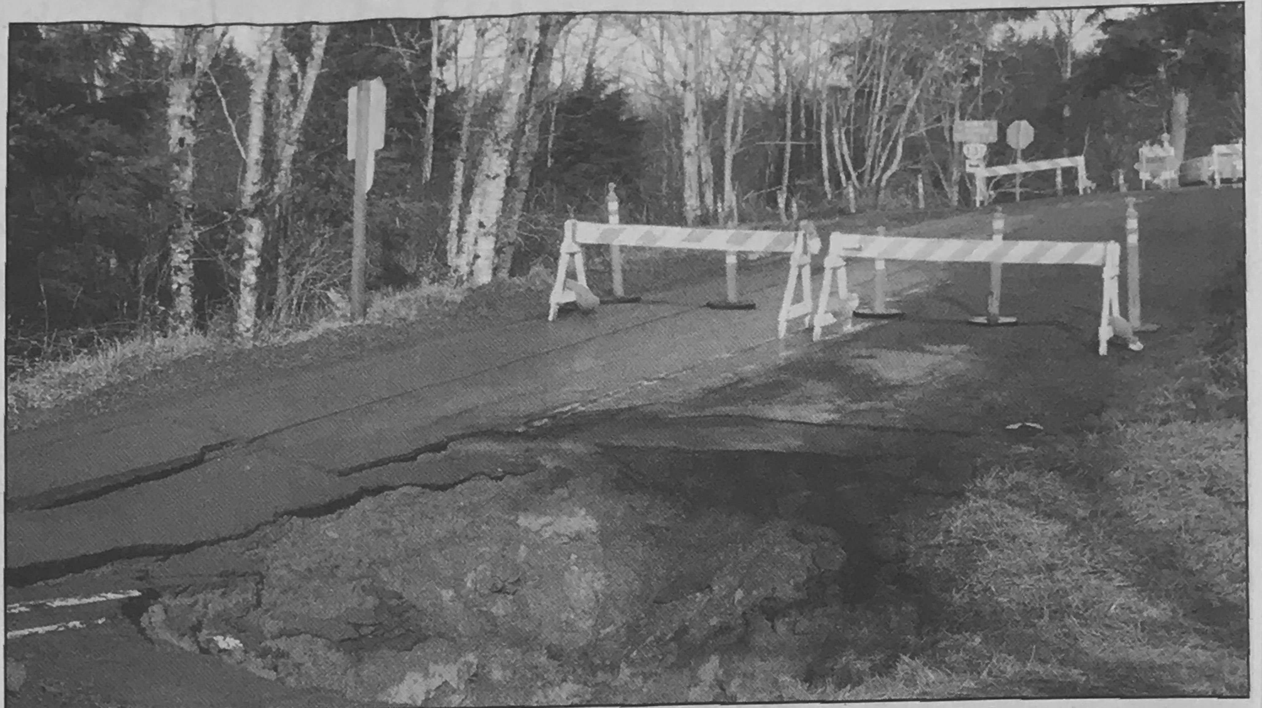
ABOVE: A sink hole caused by a culvert failure developed on Bilyeu Avenue near SR 131 in Netarts following last week's rainfall.
